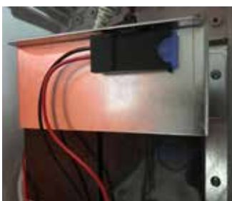
4. Unscrew the bracket holding the batteries. Remove the bracket and batteries.
