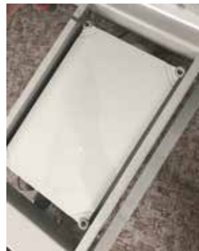
2. Unscrew the plastic lid on the battery box.
