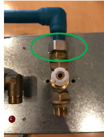
Loosen and remove the valve from the plastic pipe unit by using a spanner.
